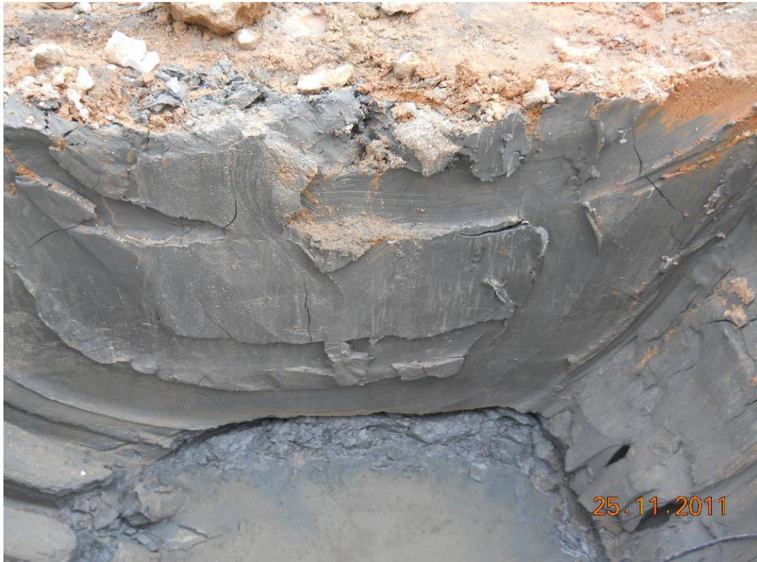
Fig. 2 Marine Mud Encountered in the Building Contract
