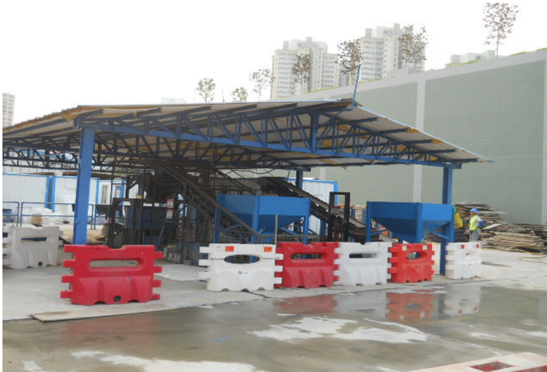
Fig. 5 Temporary Factory for Production of MMMM at Site
