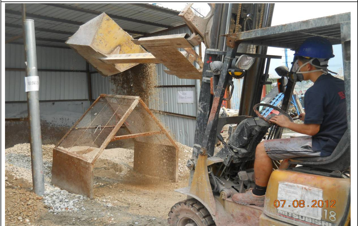
Fig. ii Sorting Recycled Aggregates
