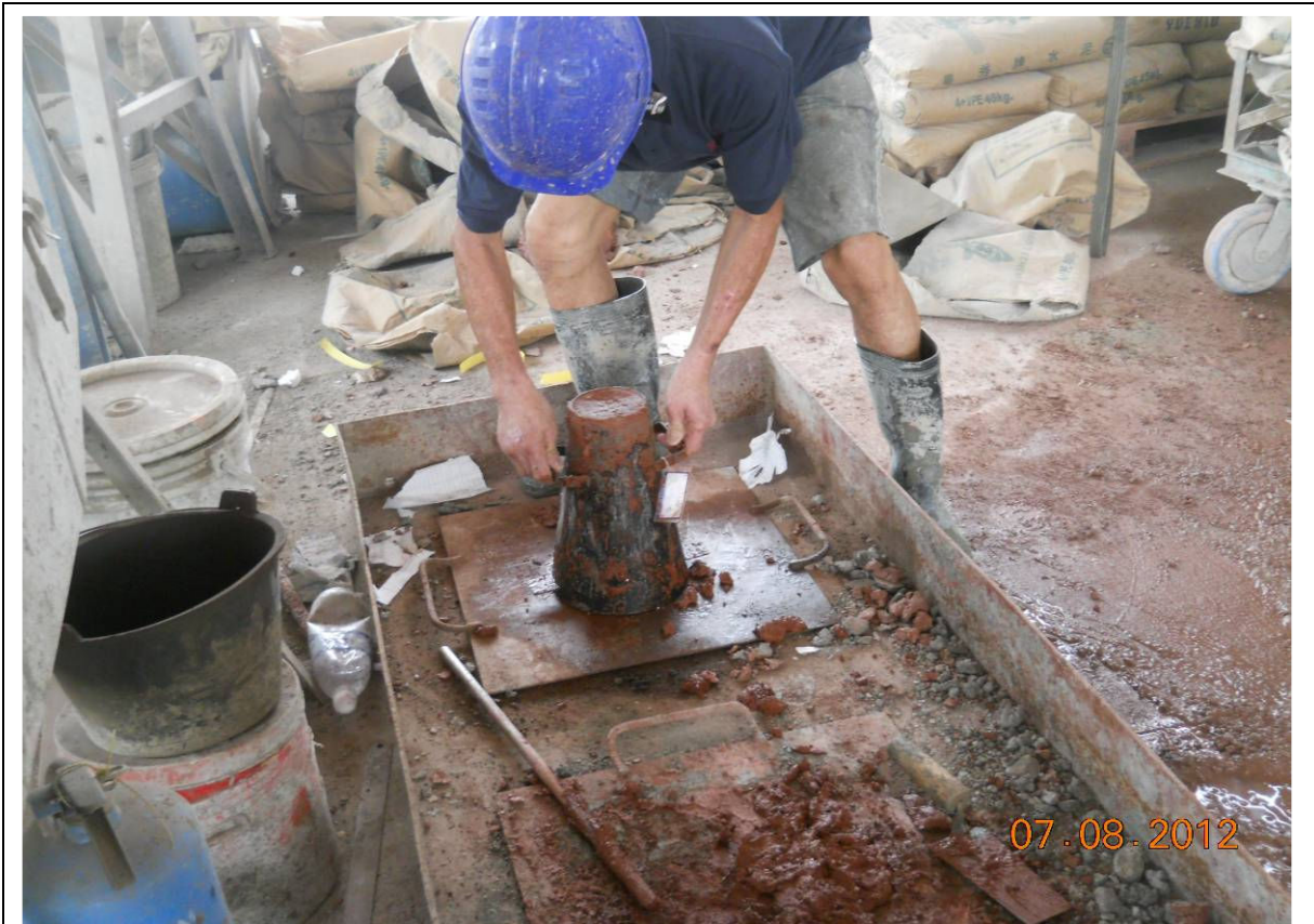
Fig. ix Conduct Slump Test to MMMM Mixture
