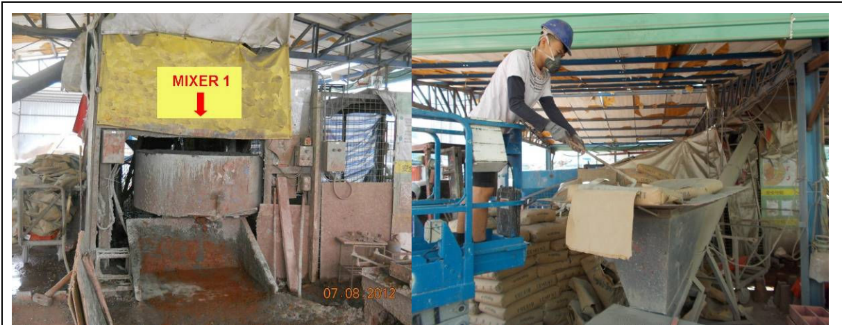
Fig. v Pre-mix Cement and Recycled Aggregates in Pan Mixer No. 1
